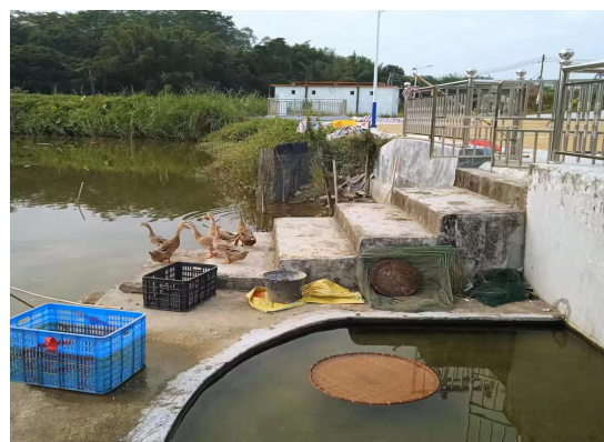
拟建挡墙栏杆现状
